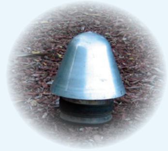
Mushroom-type backflow prevention device
