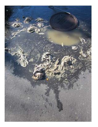
The picture above was taken after nondispersing materials clogged a local sewer main, causing sewage to overflow onto a public street. The Stege Sanitary District is committed to maintaining its sewer system and preventing overflows, however we need your help to protect the environment and keep sewage in the pipes.
